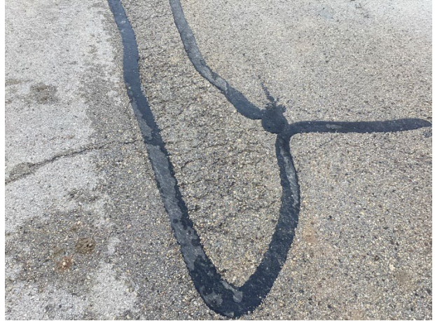
Crack repair overview
