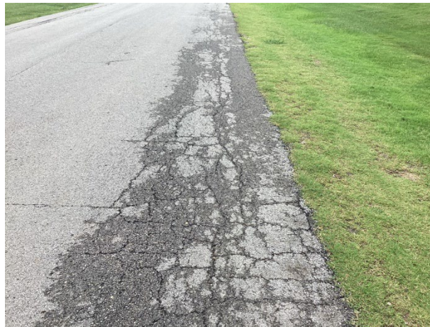
Pavement cracks at White Drive
