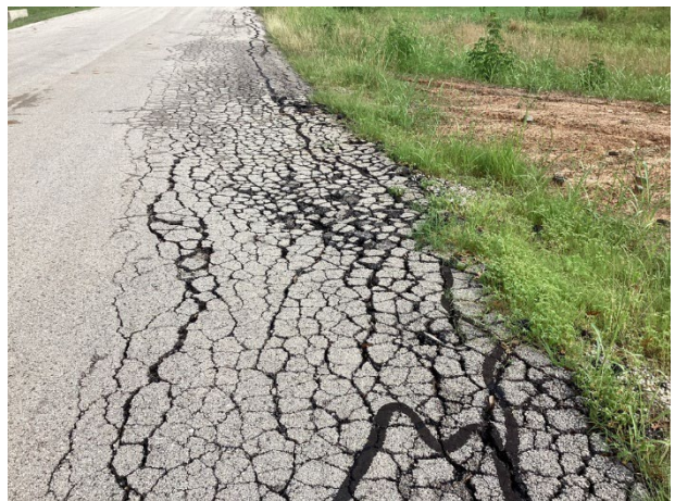
Alligator cracks at Heathington Boulevard near cul-de-sac
