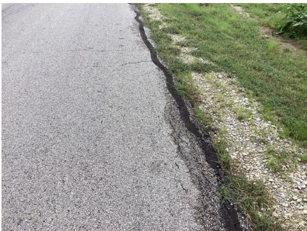
Edge deterioration at Heathington Boulevard
