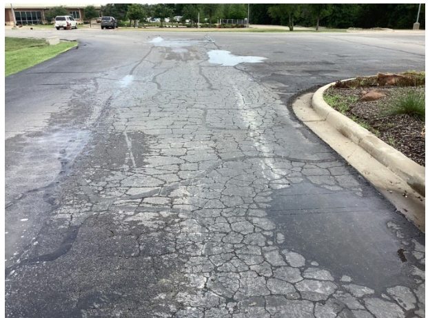
Alligator cracks and settlement at entrance
