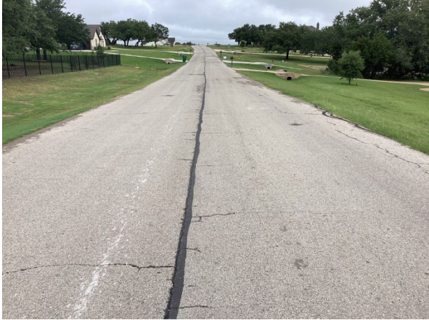
Pavement overview at Helton Drive with centerline deterioration
