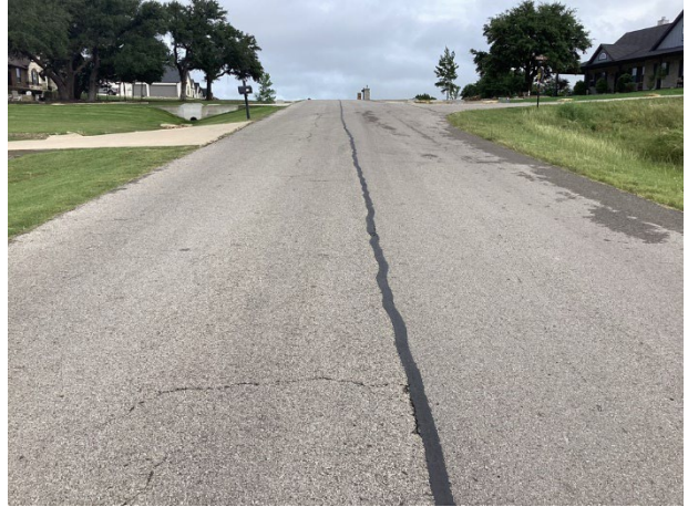
Pavement overview Martin Drive with centerline deterioration
