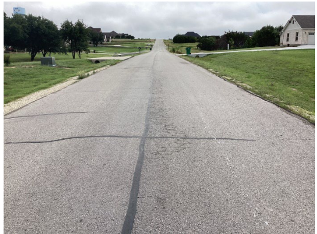
Cracks repair at Heathington Boulevard
