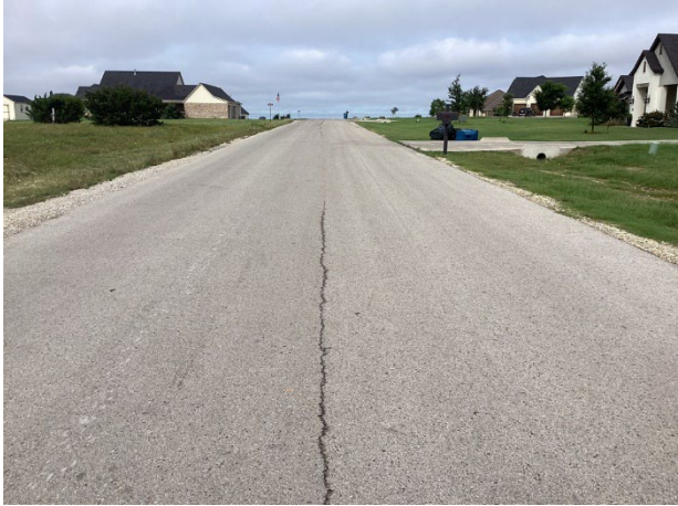
Pavement overview at Heathington Boulevard with centerline crack
