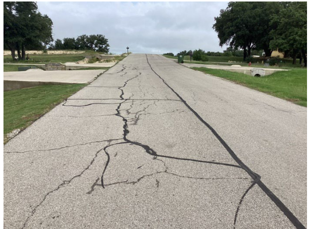
Pavement overview at Maverick Court with crack repair
