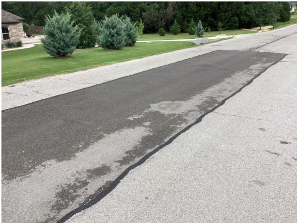
Pavement patch at Helton Drive
